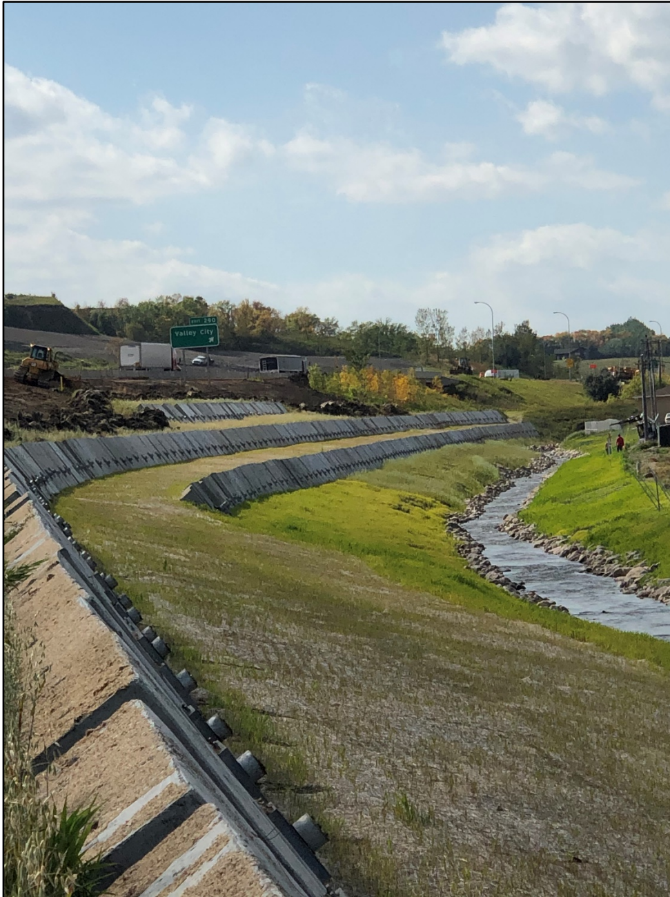
Figure 4.8.2 – Interstate 94 Between Exist 292 and 290 Landslide Repair Anchors
